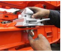
**2.** Push twist lock securing into the under mount ensuring that the handle inwards.
